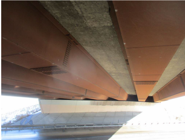
ITEM120A = SBGP: Steel Prestressed Box Girder, Simple
