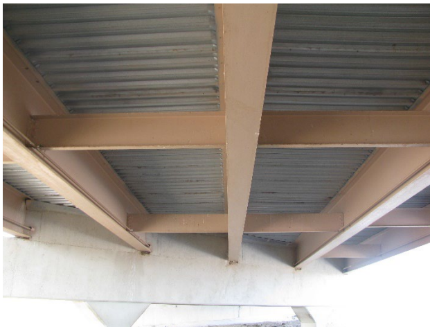
ITEM120A = CIKP: Concrete deck on Prestressed Steel I-beam, Simple
