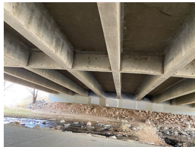
ITEM120A = CSGP: Concrete Prestressed Slab and Girder (Tee Beam), Simple
