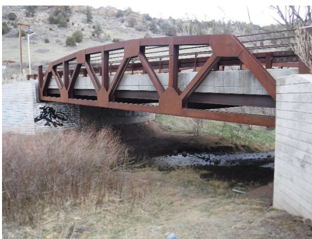
ITEM120A = SLT: Steel Low Truss, Simple
