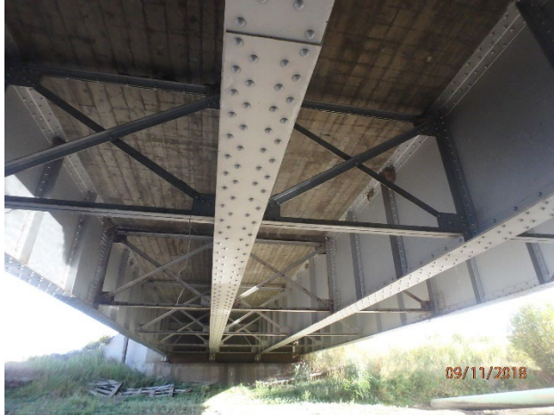
ITEM120A = RG: Riveted Girder, Simple
