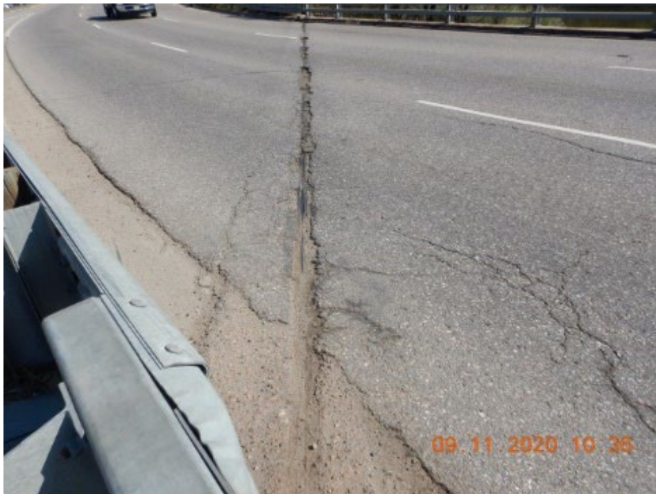
ITEM124 = B: Compression Joint Seal (elastomeric)
