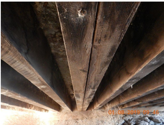
ITEM120A = TTD: Treated Timber Stringer with Concrete Deck
