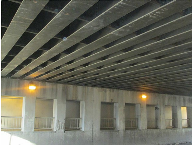
ITEM120A = CI: Concrete deck on Steel I-beam, Simple
