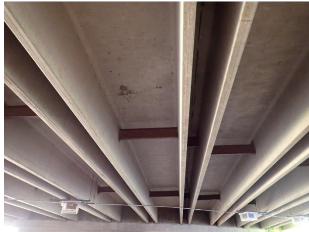
ITEM120A = CDTPG: Concrete Double T Prestressed Girder, Simple
