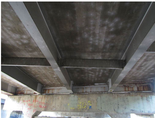
ITEM120A = CIC: Concrete deck on Steel I-Beam, Continuous
