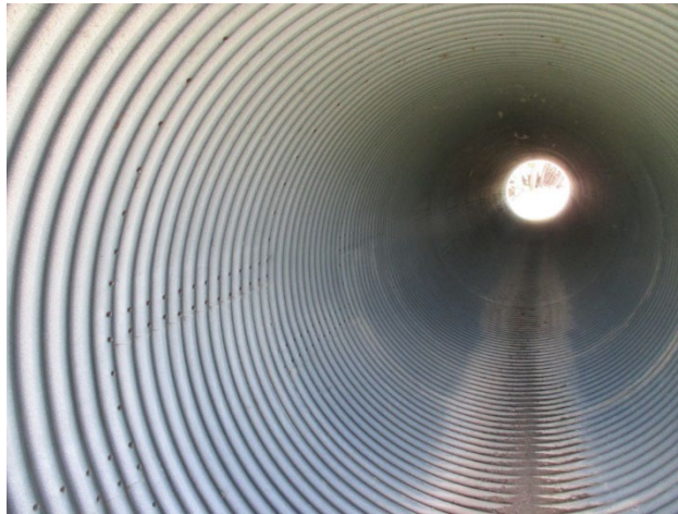
ITEM120A = CMP: Corrugated Metal Pipe Culvert
